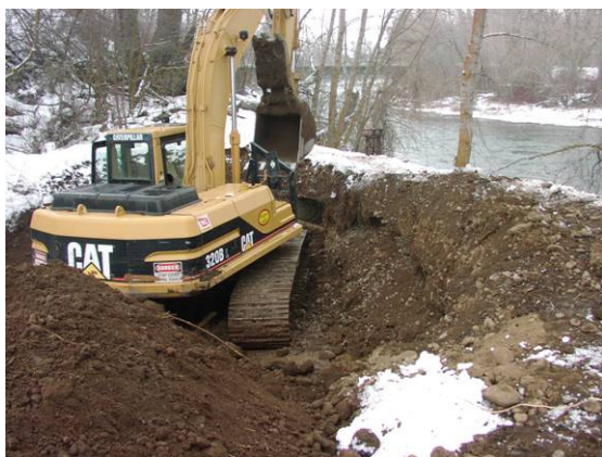
Contractor replacing inlet culvert to Fogarty Ditch, February 2007.
