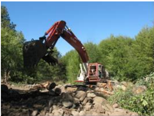
Excavator placing logs on Swale Creek, 2008.
